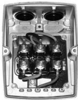
Figure 5.9 Terminal box of an asynchronous motor
