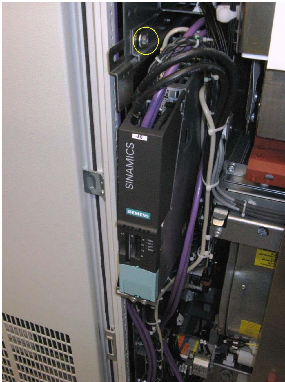
Fig. 2: Removing the CU320 with support plate
