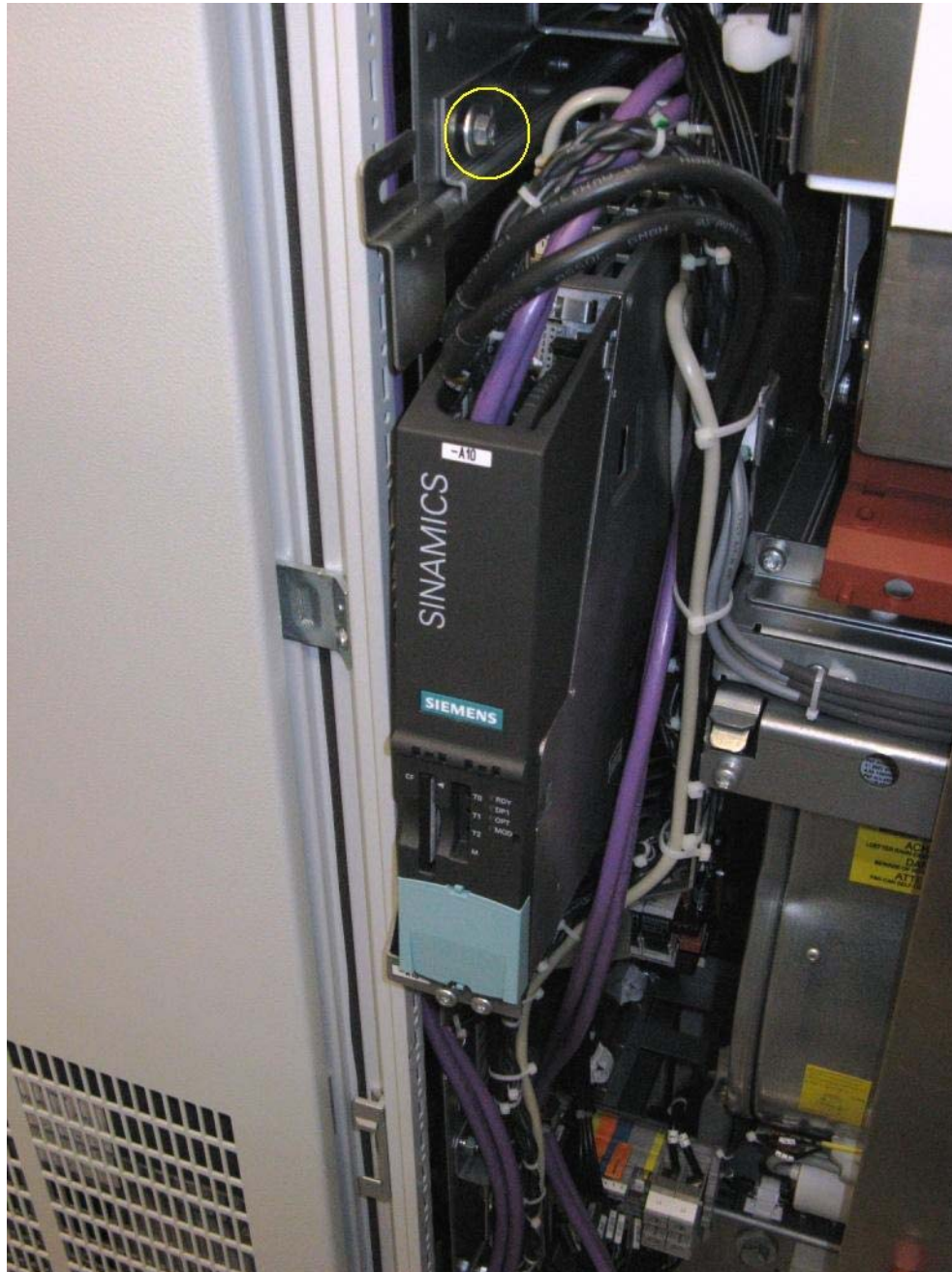
Fig. 2: Removing the CU320 with support plate
