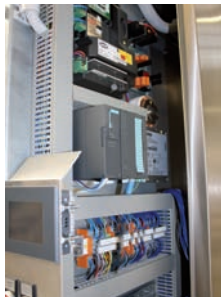
Section 2 - Zone 2 is where all electronics (e. g. PLC for measurement and counter for payment) are located, with an intrinsically safe cable connecting Zones 1 and 2. Siflow FCO70 Ex CT has an integrated barrier and requires no further Ex barrier investment.
